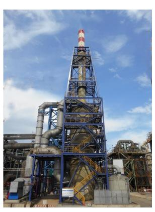
Pic. 12: SUPER<sup>OX</sup>-Process downstream sulphuric acid plants
