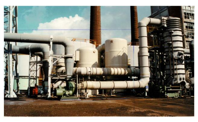
Pic. 6: Scrubbing plant for the absorption of noxious gas components and the removal of acidic mists and salt aerosols downstream of multiple-hearth furnaces for the production of inorganic raw chemicals
